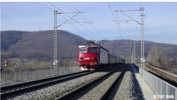
Modernisation of the main railway stations in Romania
