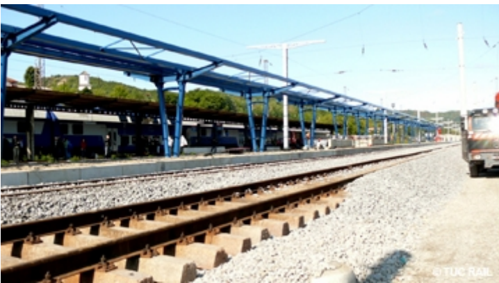
Modernisation and upgrading of the Bucharest - Brasov railway line in Romania
