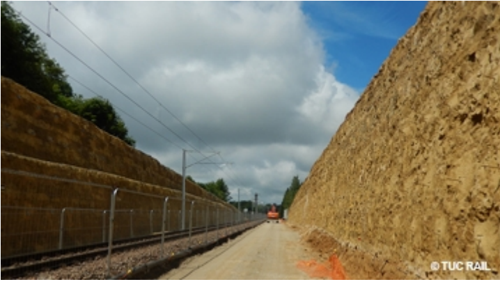
Modernisation and upgrading of the Campina-Predeal railway line in Romania
